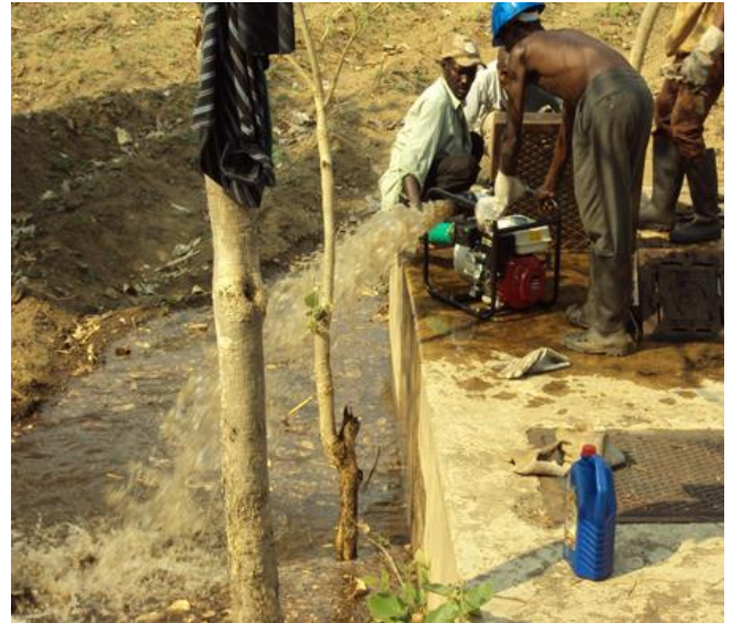
7B: Emptying water from chamber for maintenance
