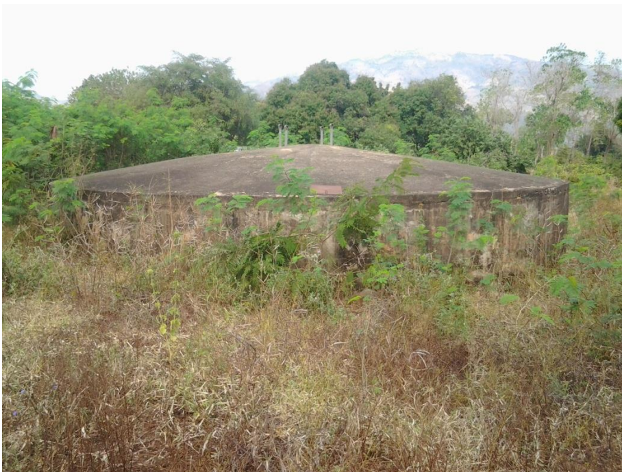
Figure 15: Water Storage Tank in EBWSS
