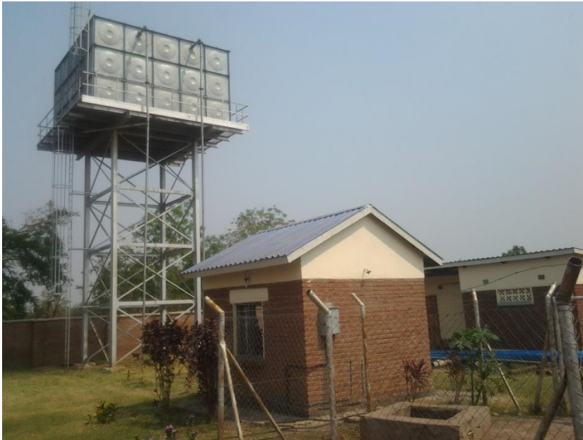
Figure 10: A Water Storage Tank at MFWSS
