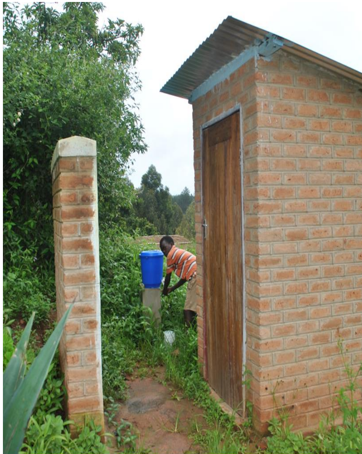
Figure 7: An Improved Pit Latrine
