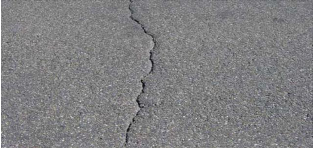
Figure 2.4: Cracking
