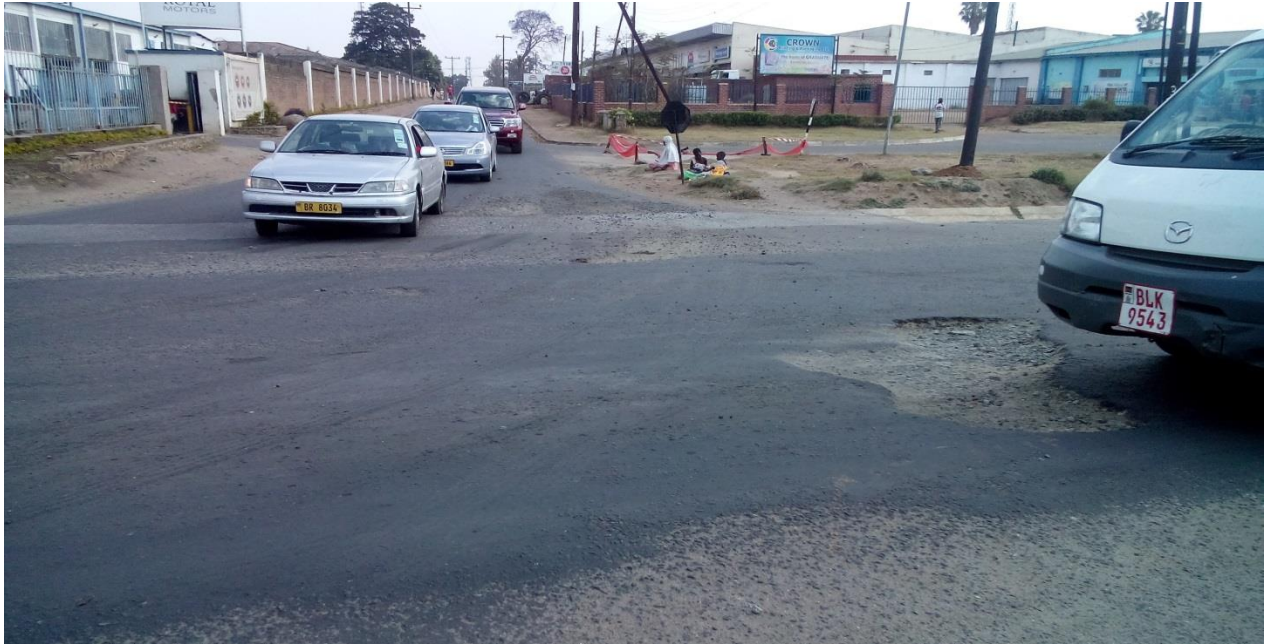
Figure 1:3: Part of Newly Constructed Blantyre-Zomba Road (Limbe Section)
