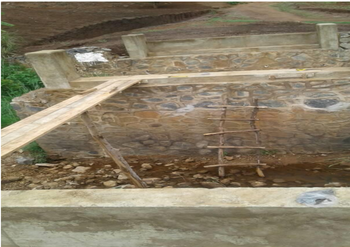
Figure 4.4: Nasundu Bridge New Concrete Caps
