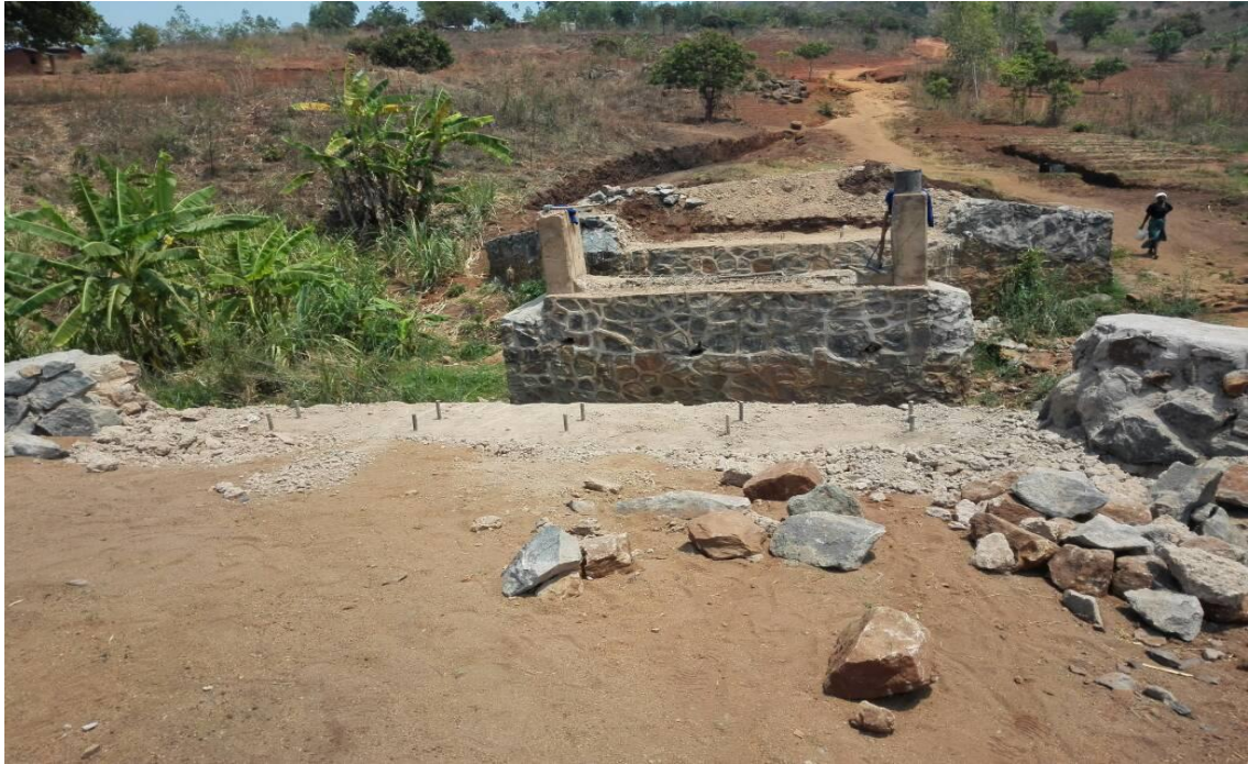
Figure 4.3: Demolition of Nasundu Bridge Concrete Caps
