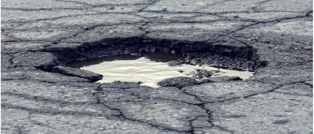
Figure 2.5: Pothole
